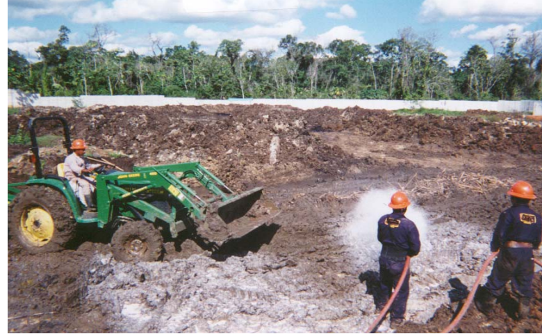
Fig. 2 SuperAll/Water (1:8) application
