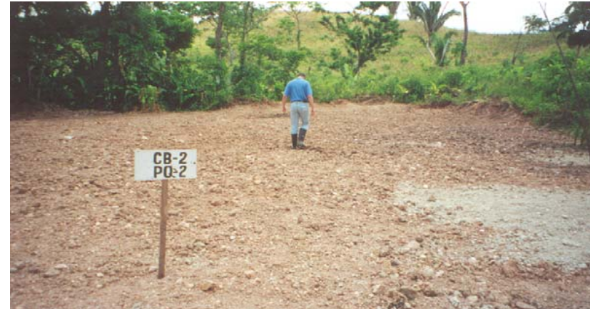
Fig. 4 Pit backfilled - (6 months)
