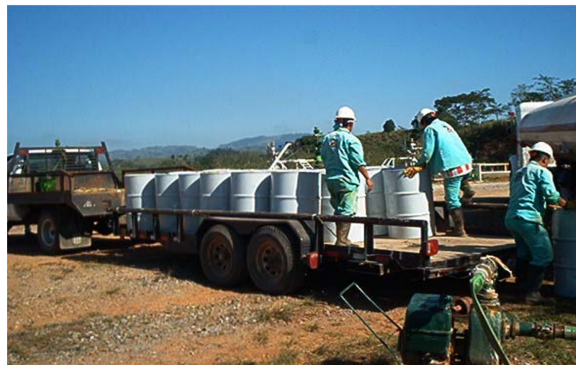
Fig. 2 Diluting SuperAll#38 in tank truck with water (1:8)
